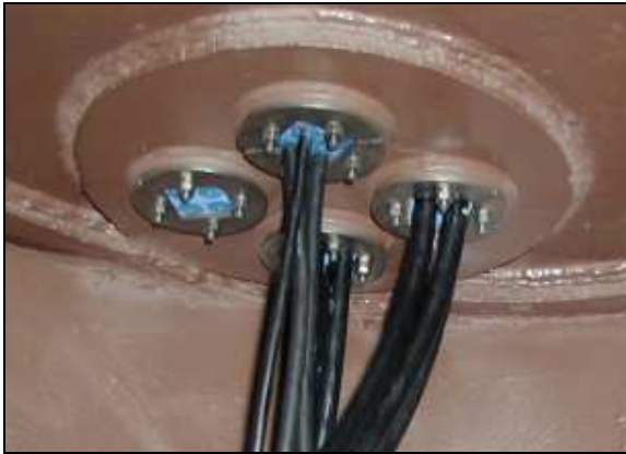
Figure 7c – Cable Pipe No. 3
