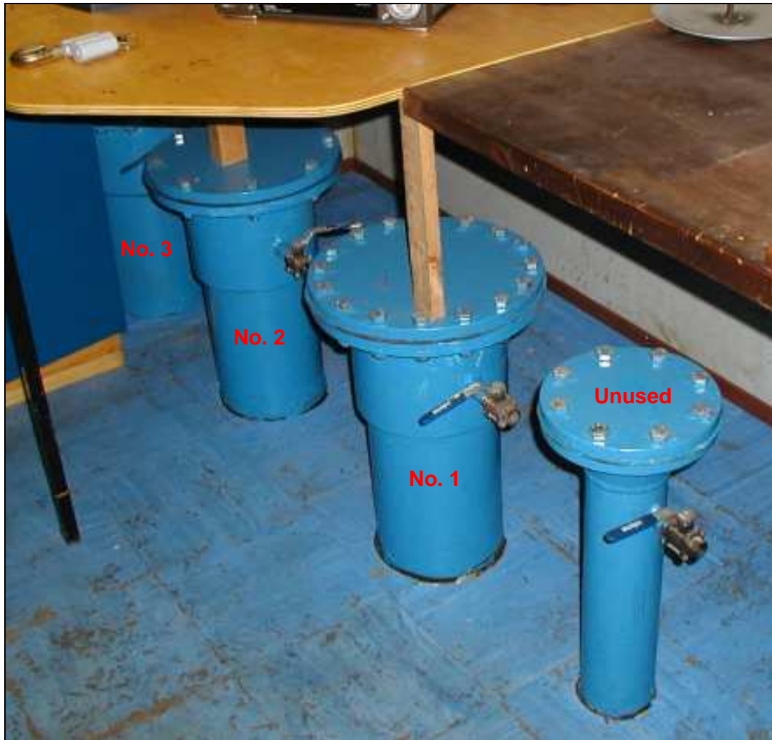
Figure 5 – Cable Pipes Prior to Installation
