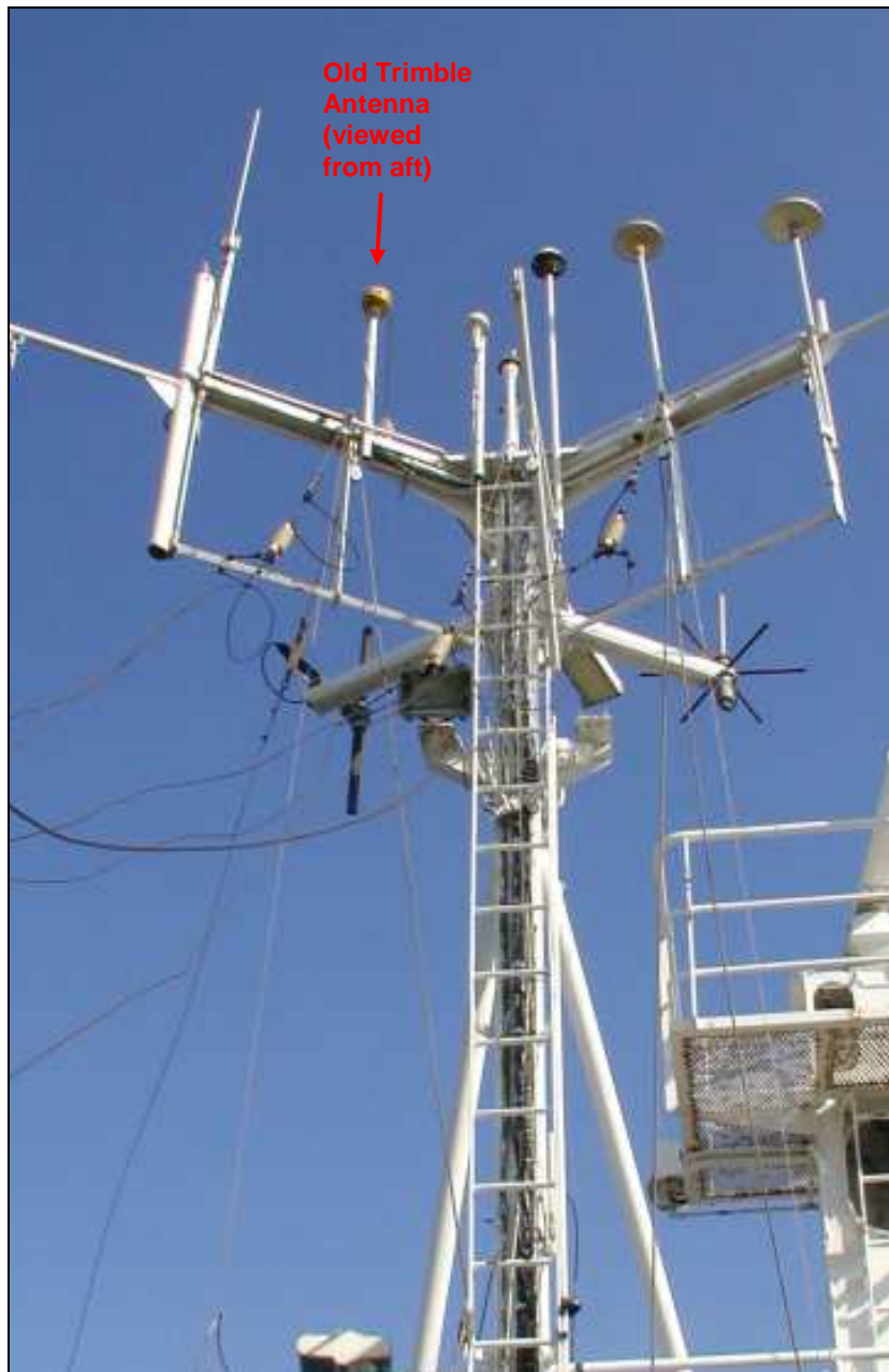
Figure 20 – GPS Antenna Installation
