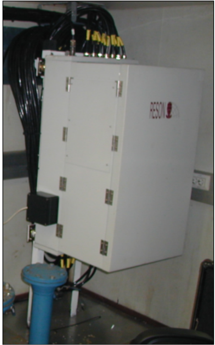
Figure 17b – Transceiver Installation
