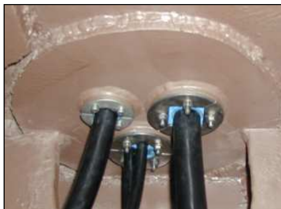
Figure 7b – Cable Pipe No. 2
