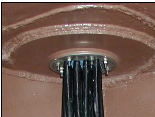
Figure 7a – Cable Pipe No. 1
