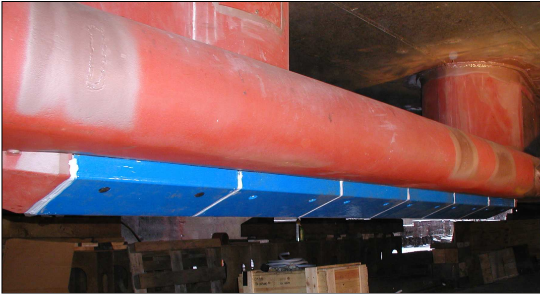
Figure 9 – SeaBat 8150 Transmitter Installation and Sealing
