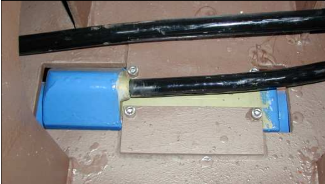
Figure 11a – 8111 Transmitter Installation
